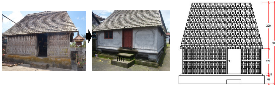
Figure 1. The building dimension of Bali Aga dwellings tends to be small with a very small proportion of opening. (a) Dwellings with the concept of Bali Aga in the initial period (b) Bali Aga dwellings that have been affected with modernization. (c) Proportion dimension of the opening hole towards of the wall
