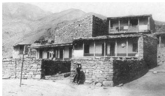
Figure (3), Model of Circassian house. A row of rooms adjacent longitudinally in front of it open Balcony slightly elevated approximately 50-70 cm above the balcony is an extension of the roof of the rooms, supported by a number of strong wood sticks.
