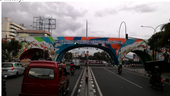
Figure 1.1 sample of path in Bandung City Picture of "Pelangi" overpass from the north side.
