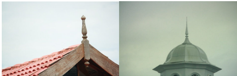
Figure 14: Application of tunjuk langit
