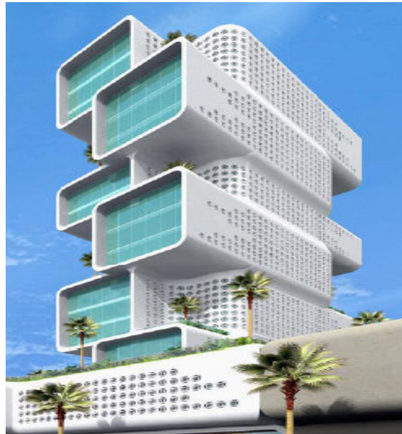
Plate 6: Showing an Apartment building constructed with a lightweight concrete Source: Robyn.G (2008)
