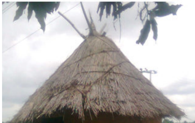
Plate 11: Grass used a material for Roofing Author's fieldwork.2011
