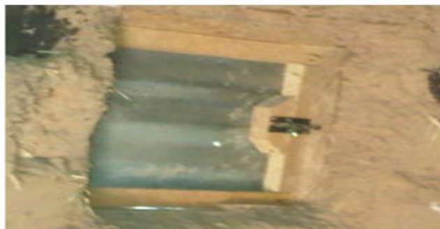
Plate 10: A window made up of wood and Zinc. Author's fieldwork.2011
