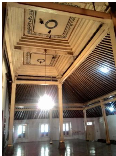
Picture 5. Appearance of Saka guru on the Interior of dalem Sasana Mulya (Photo: Documentation by Siti Badriyah, 2016)
