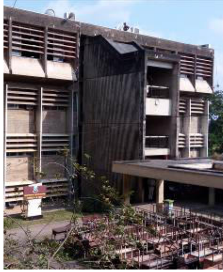
Plate 5: Drilled parapet walls for AC piping (Source: Author, 2016)
