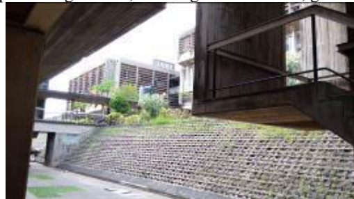
Plate 2: Concrete retaining walls with basket weave appearance perforations (Source: Author, 2016)
