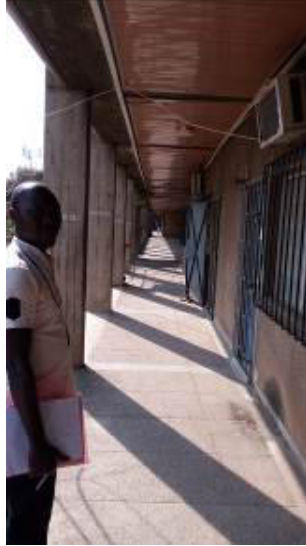
Plate 4: ceiling replaced with PVC panels (Source: Author, 2016)
