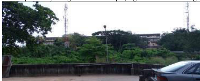
Plate 1: North approach view (Source: Author, 2016)
