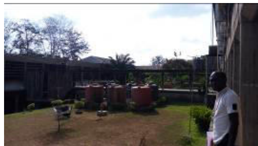
Plate 3: Courtyard area encroached upon with unguided intrusion of some services (Source: Author, 2016)
