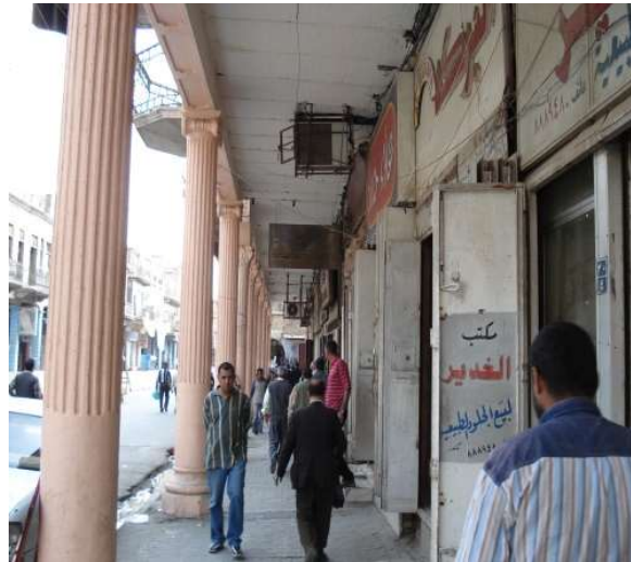
Picture No. (2) Explains the relationship of Setback and building coverage with Al-Rashid Street – Baghdad
