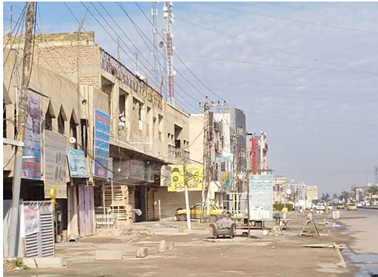
Picture No. (4) Shows the relationship of the buildings with the sidewalk on Baghdad Street, after changing the legislation
