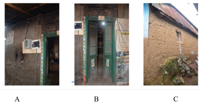
Figure 5. Opening space in Raras' bale gedé saka roras tumpang talu in Sidatapa village, in the form of ventilation holes (a), door holes (b) on front façade, and window holes in side façade (Maharani, 2018)
