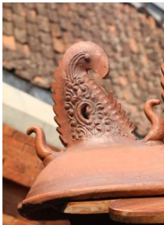
Figure 4. Wuwung Ornamental Art Placed at the Top or Bottom Corner as a Lock or Placed at the Most Corner in the Traditional House Kudus “Wuwungan Bulusan” (Photo Suharson, May 15, 2020)
