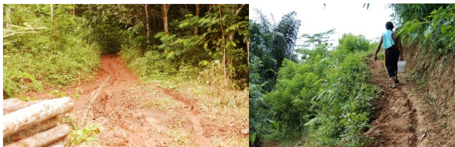
Figure 4. Observation of road conditions in Cikadu
