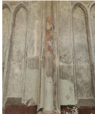
Figure 9. Wall Restoration Process Santa Ursula Chapel
