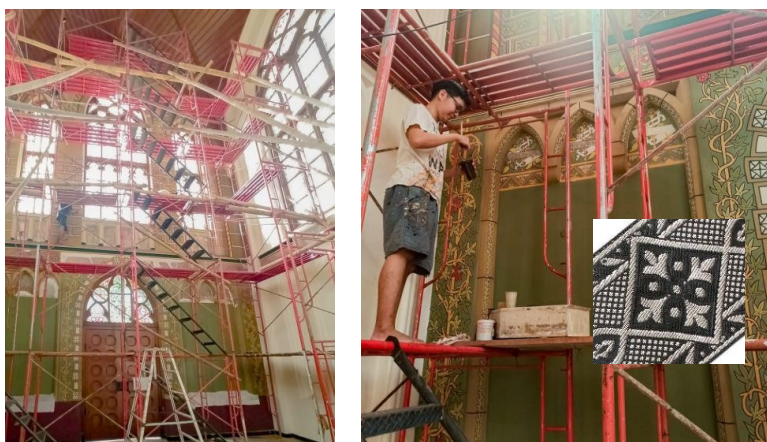
Figure 11. Wall Mural Restoration at Santa Ursula Chapel
