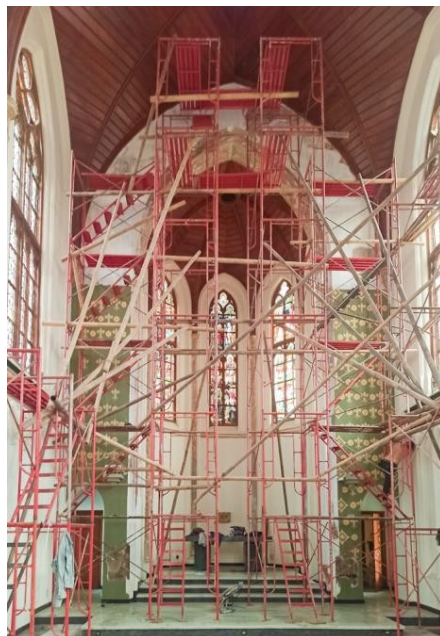
Figure 4. Restoration Process - Santa Ursula Chapel (Phase 3)
