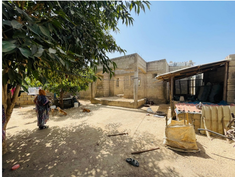
Figure 1, Uncompleted Building used as temporary Shelter , Image by Female FGD Group A, February 2024, Sabon-Gari Community of Resettled Persons, Maiduguri-Borno state, Nigeria.
