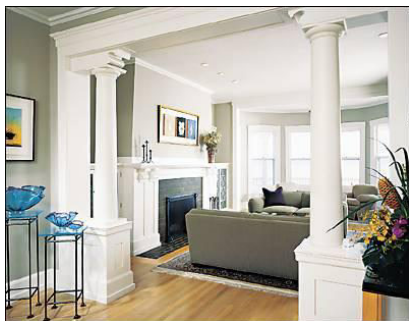
13: Using non supporting Tuscan gypsum columns to divide space.
