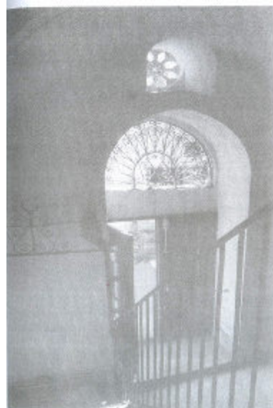
Picture (7) the main entrance to the building of Toukan.
