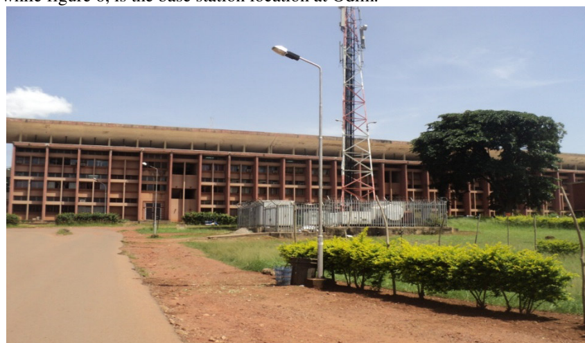
Figure 5 Base Station located at the faculty of Arts
