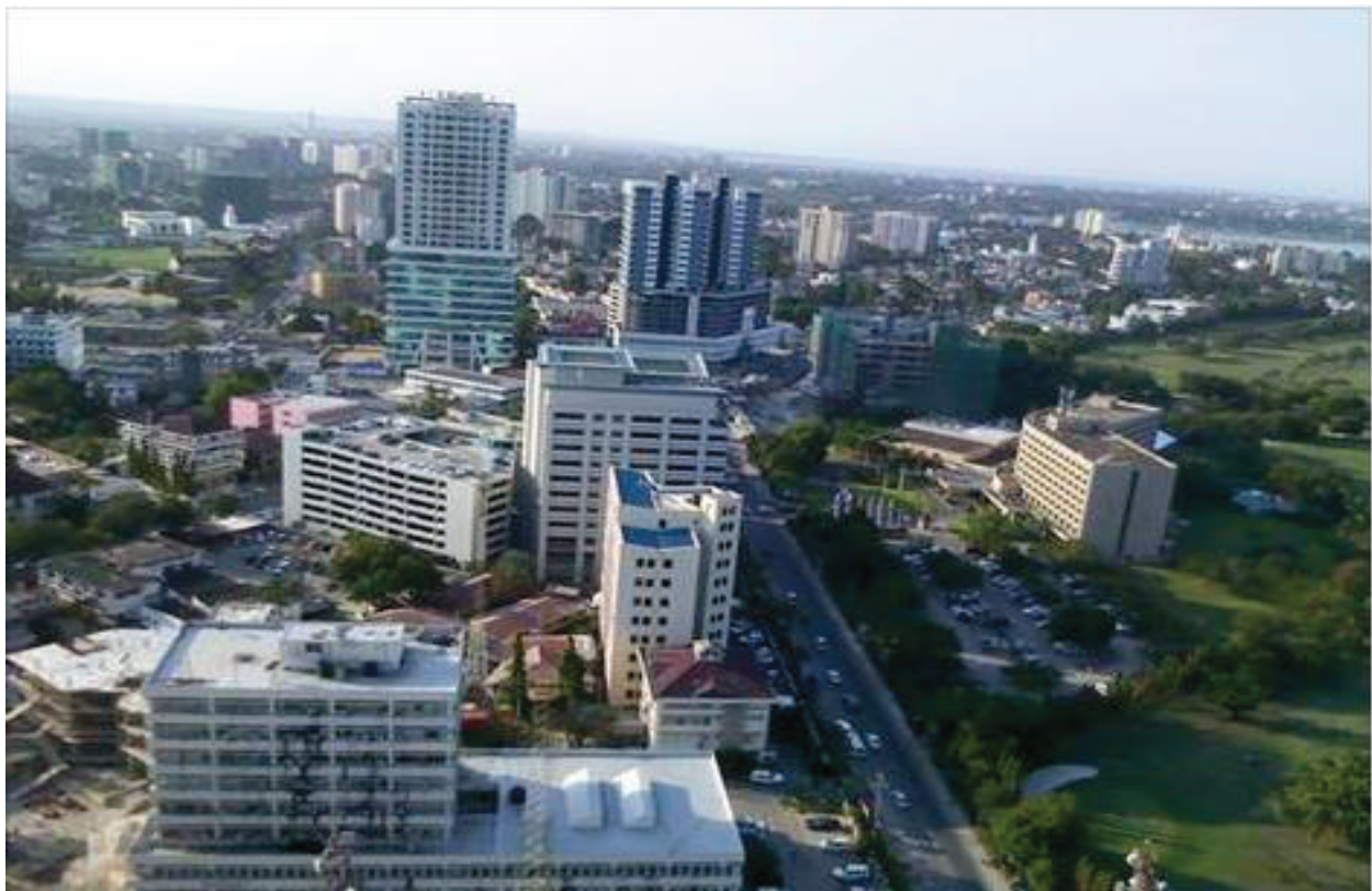
Figure 2: Diagram showing some tall buildings in Dar es Salaam as viewed from Posta PPF house
