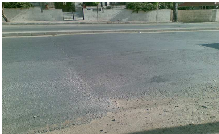
Fig. 2. Invisible speed inhibitor due to the deficiency of paint or light reflectors usage
