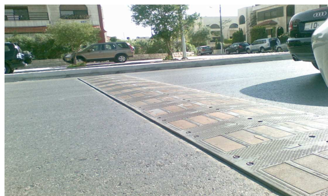
Fig. 3. Modern speed inhibitor made of rubber and springs
