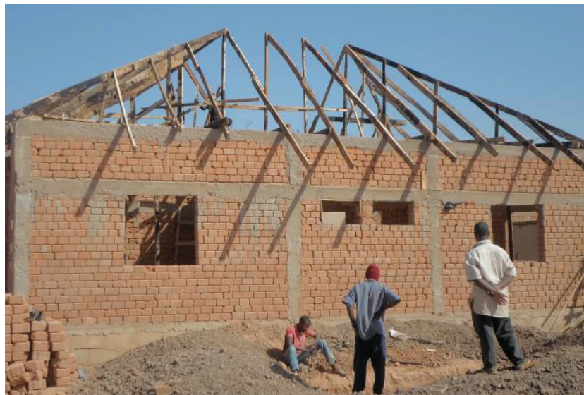
Fig. 2. Hydraform Building under Construction
