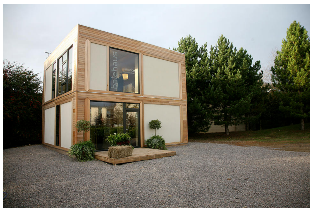
Fig.4: The BaleHaus experimental building at Bath
