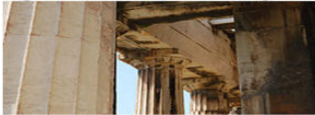
Temple of Hephaestos, fluted Doric columns with abacuses supporting double beams of the architrave
