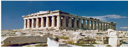
The Parthenon, shows the common structural features of Ancient Greek architecture: crepidoma, columns, entablature, pediment.
