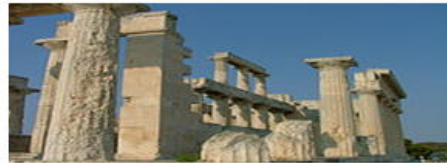
At the Temple of Aphaia the hypostyle columns rise in two tiers, to a height greater than the walls, to support a roof without struts.
