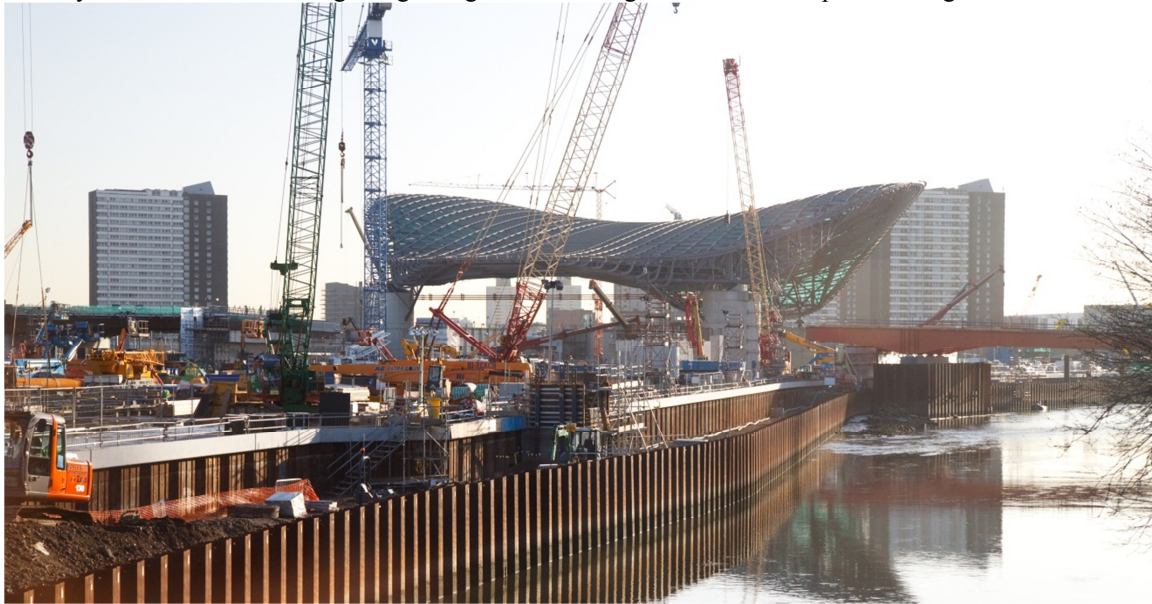
Figure 3. During the construction process
