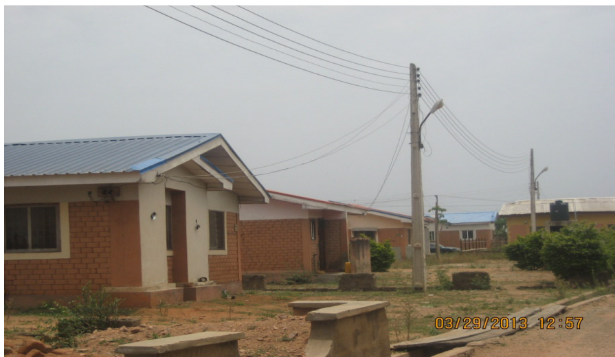
Plate 2: Houses constructed with Burnt brick
