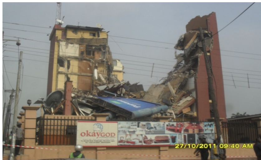
Figure 8: Collapse site of a multi storey building in Lagos, State, Nigeria.
