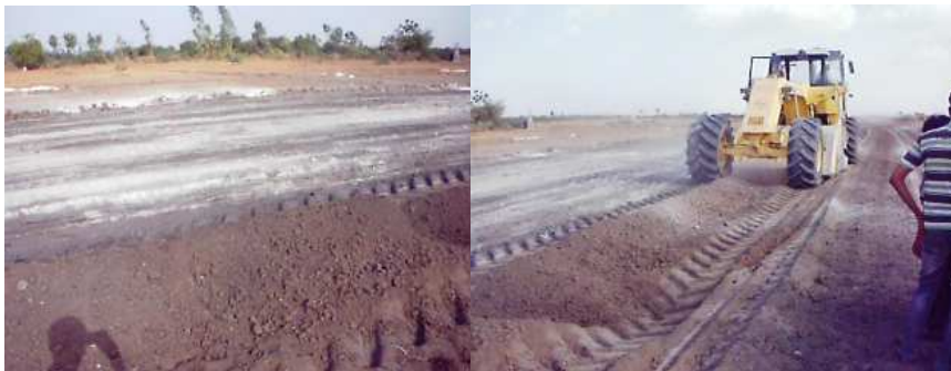
Fig. 1 Laying of fly ash/lime on subgrade soil Fig. 2 Onsite mixing machine
