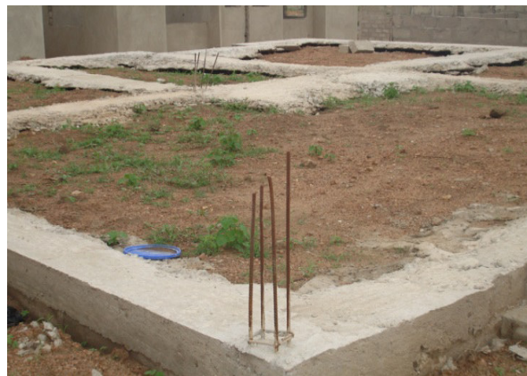
Plate 8: A Type of Oversight Concrete Method (“German Concrete”) Used at Most Sites
