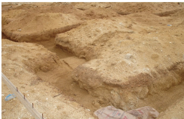
Plate 1: Depth of Foundation Trench at some sites
