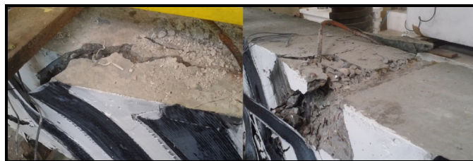
Figure 14. Cracks on the Top Surface of Beam Specimens
