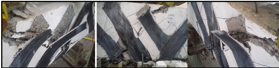
Figure 16. Debonding and Rupture of CFRP for Beam Specimen (SCC-R3-45°)
