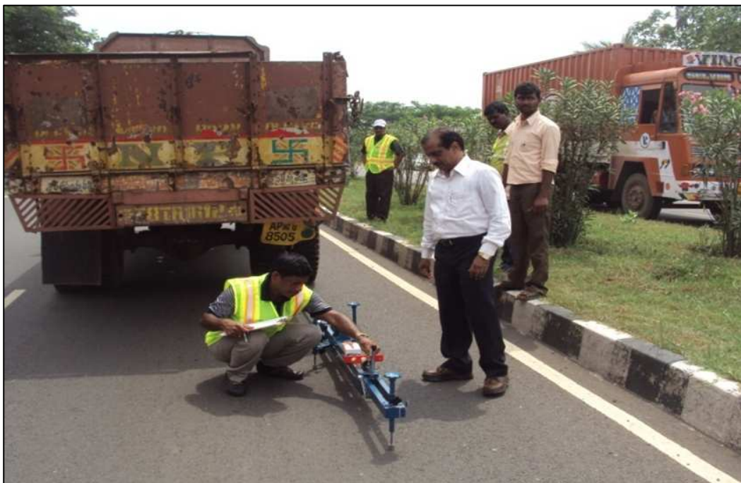
Fig: 3 Benkelman Beam Deflection Test.
