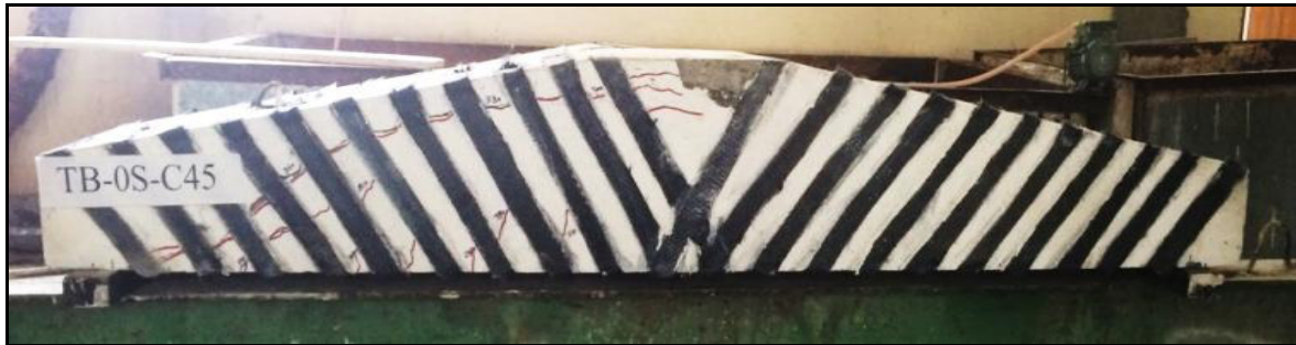
Plate 8. Crack Pattern for Beam Specimen (TB-0S-C45°)
