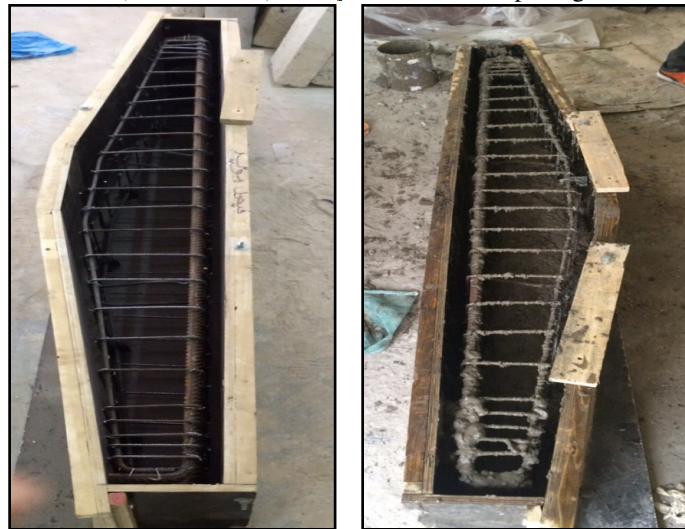
Plate 2. (a) Putting Steel Reinforcement Cage in Mold (b) Beam Specimens Casting
