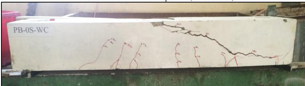
Plate 10. Crack Pattern for Beam Specimen (PB-0S-WC)
