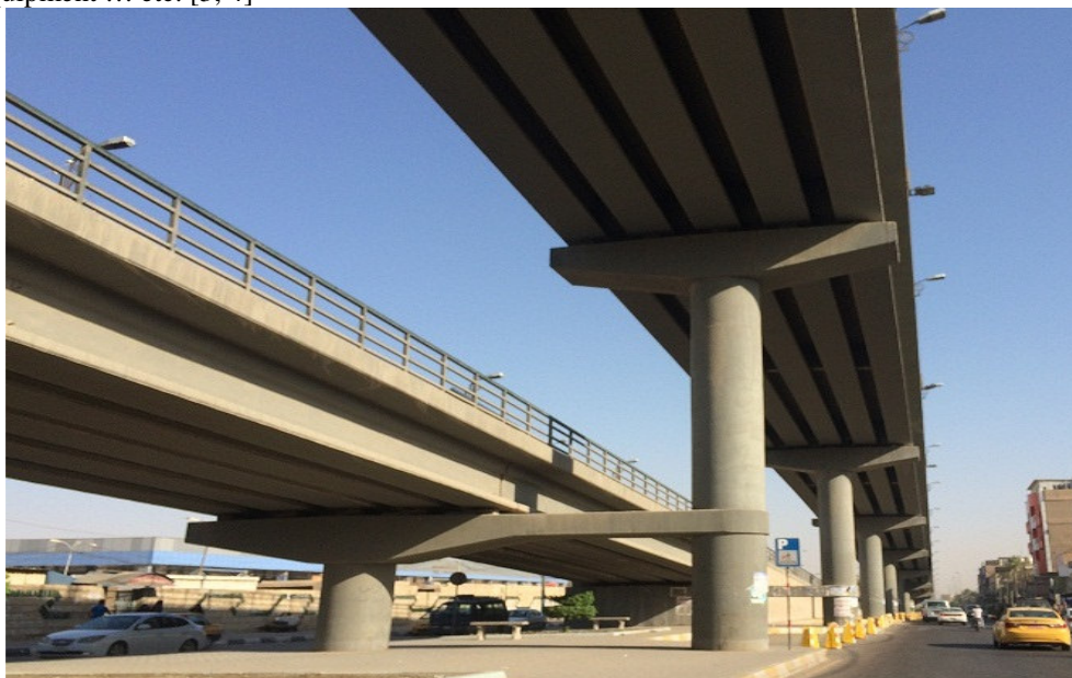
Plate 1. Thawrat Al Eshreen Bridge in Iraq.
