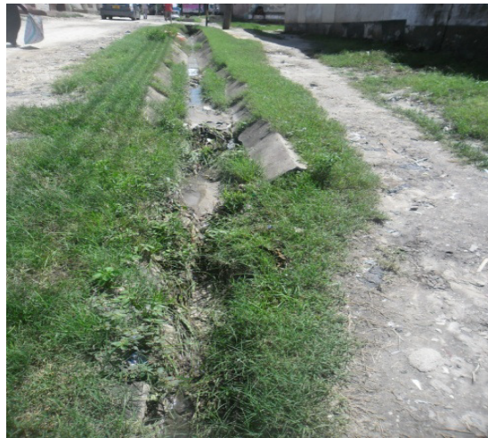
Figure 8: Condition of storm water drainage system
