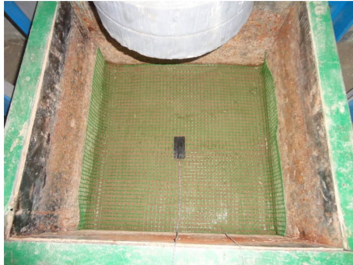
Figure 7. Place HDPE Geogrid layer above Subgrade Layer.
