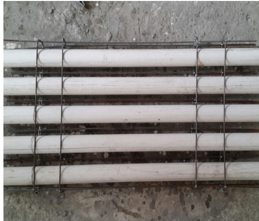
Figure 2. Steel reinforcement cage with PVC pipes
