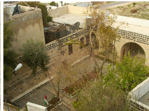
Fig.11, The renovated house
