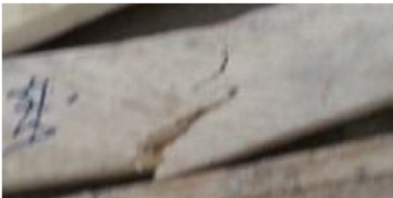
Plate 5: Bending failure in solid beam
