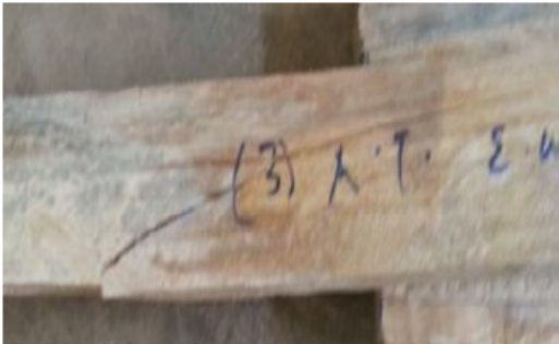
Plate 1: Bending failure in solid beam
