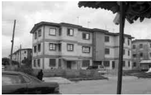
Plate 1: Entrance canopy, perimeter dwarf fence wall, car park, change of window materials
