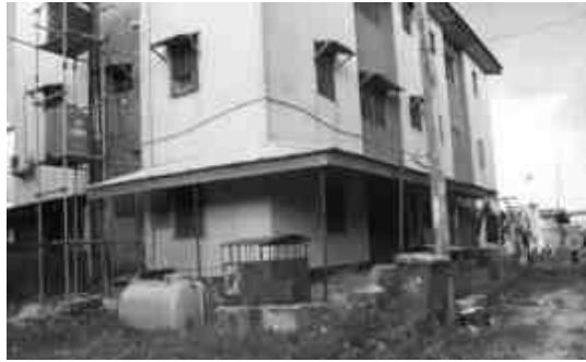
Plate 4: Covered terrace, scaffold-supported water tanks, AC unit on walls, and bedroom converted into Home-based enterprise (HBE) in Iponri Housing Estate
