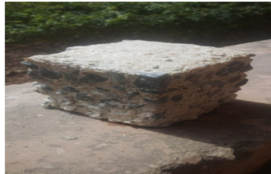
Fig3: The effect of Sulphuric acid on concrete
