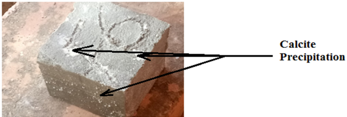
Figure 4: Precipitate on surface of concrete
