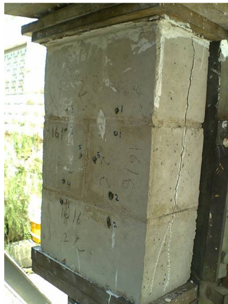
Figure 2. A tested prism built with construction method 2 with strain measurements.
