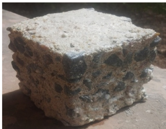
Figure 4: The effect of Sulphuric acid on concrete
