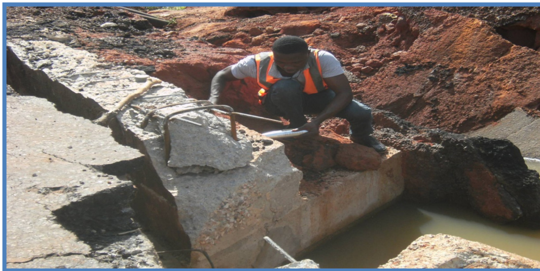
Plate 5: Concrete strength test using rebound hammer device
