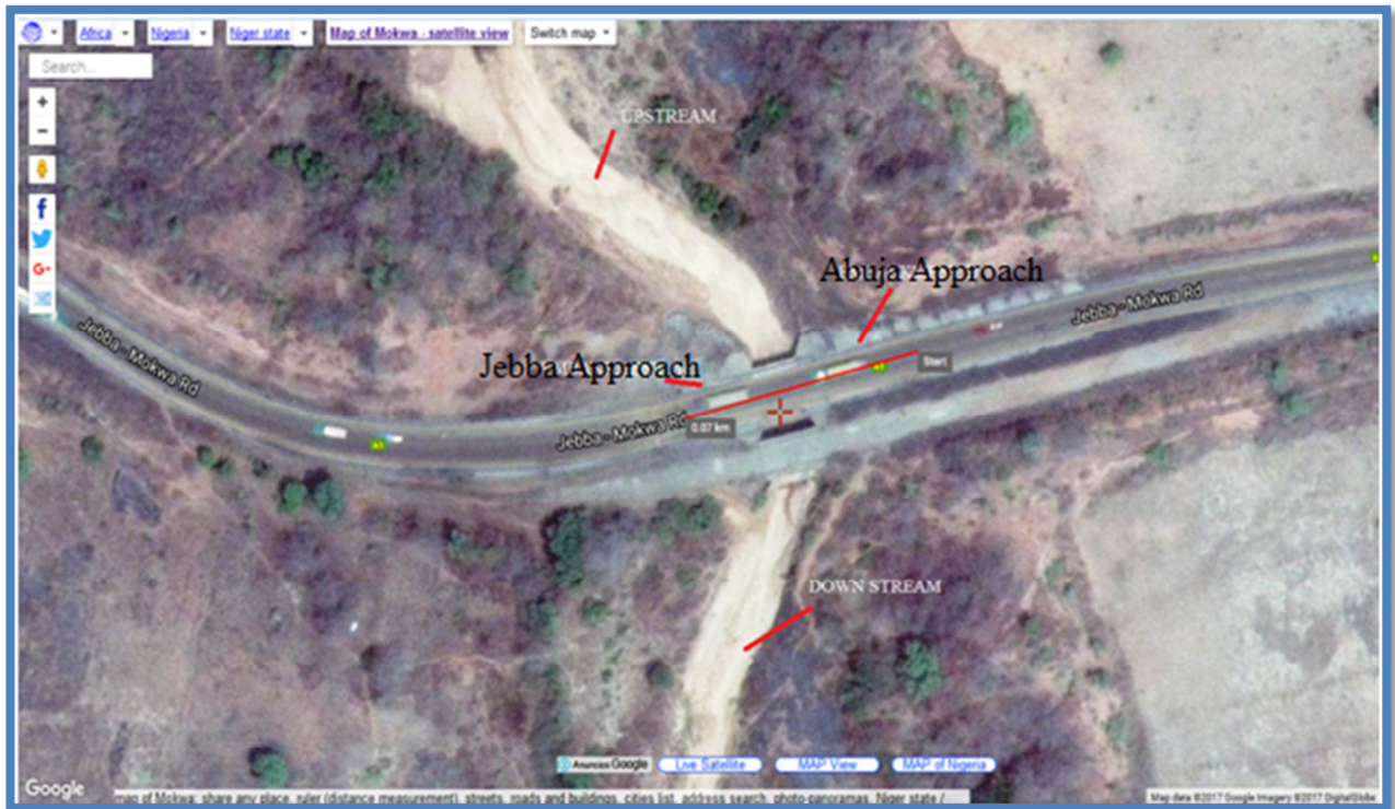
Figure 1: Satellite Imagery of collapsed Tatabu (Mokwa) bridge
