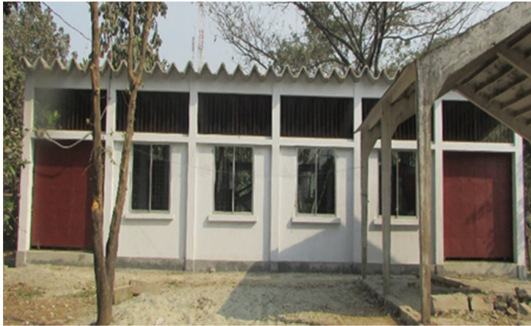
Figure03: Pilot plant shed structure for Compressed Stabilized Earth Block (CSEB) production at HBRI campus
