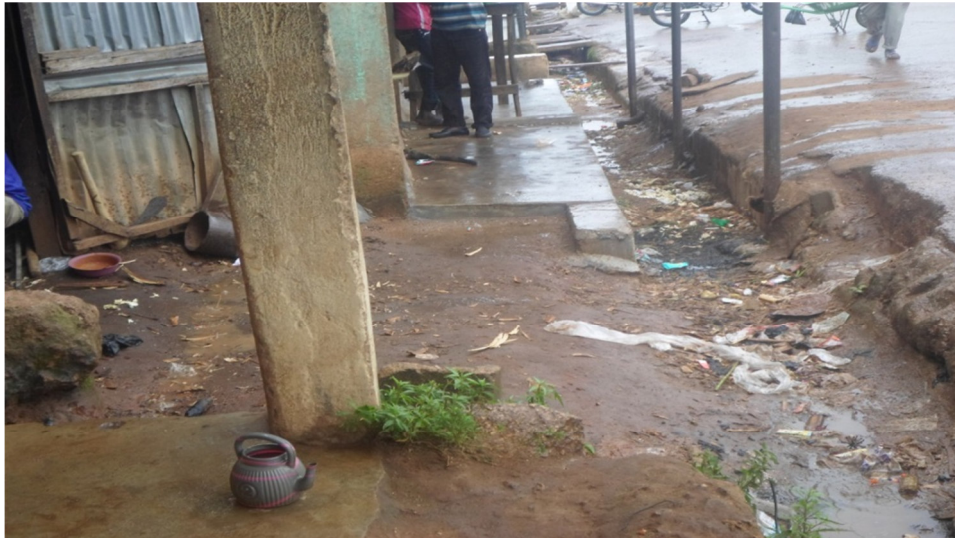
Plate 1: Blocked drainage from informal sector activity
