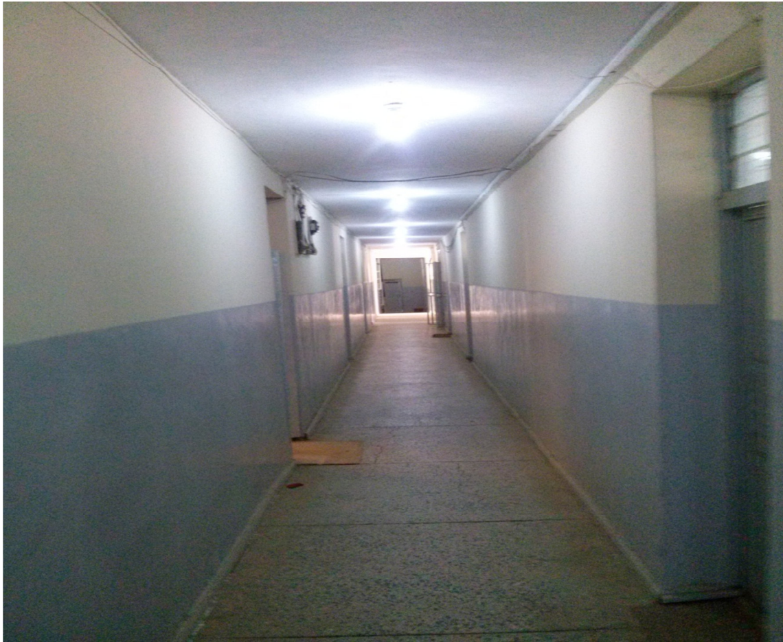
Fig 5: Typical Double-loaded Corridor in Building ID UJ ADMIN.
