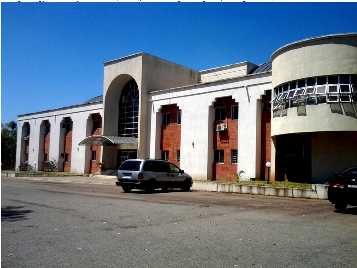
Fig 1: Typical Administrative Building Studied (Building ID: NIPSS ADMIN).
