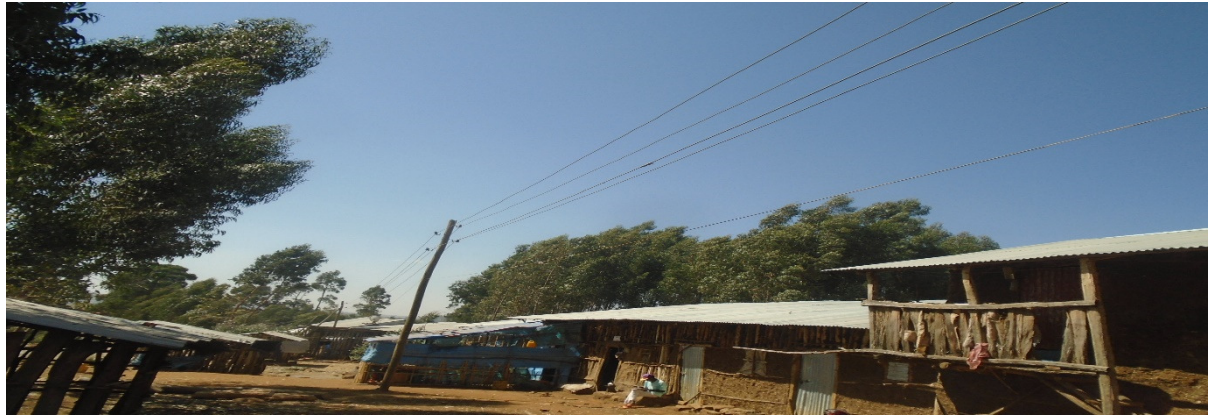
Figure 5 show hydroelectric power along the project kebles
