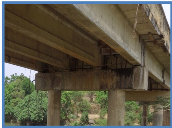
Figure 15. Formwork observed under deck.
