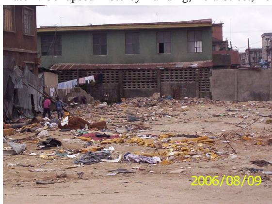
Plate 2: Collapsed 2-Storey Building, Bola Street, Ebute Meta, Lagos.
