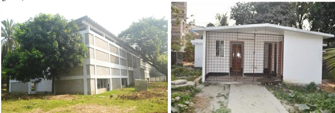
Figure 3: Display Centre (left) and Community Kitchen with Toilet by using FC Sandwich Panel (right)
