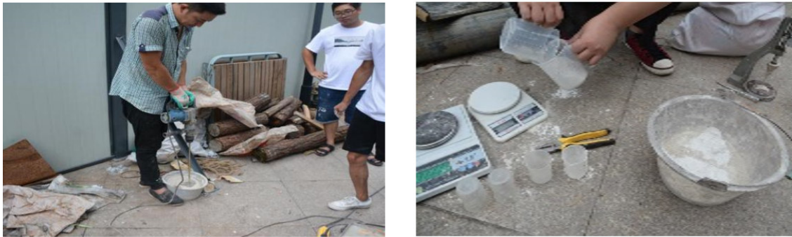
Figure 3 Site Material Preparation
