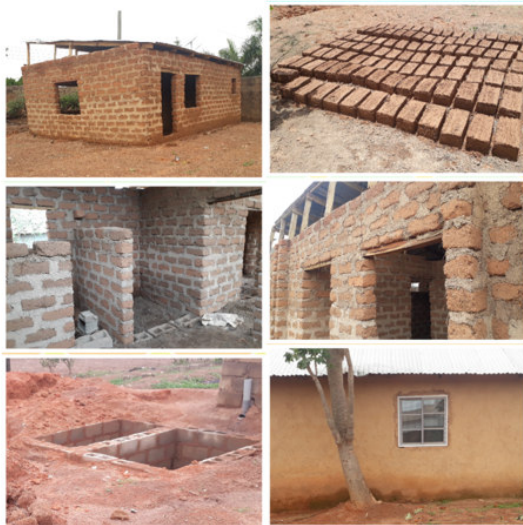
Figure 3: Low cost methods of construction using dried earth building bricks, rough-hewn wood supports, exterior finishing, underground cesspit, interior partitions (clockwise from top left).
