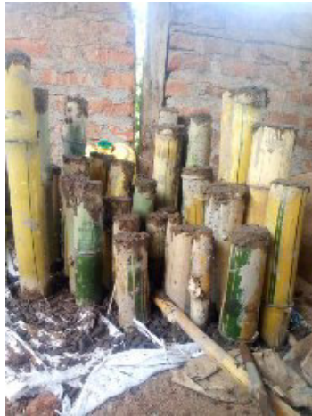
Fig 2(a) Casting of bamboo
